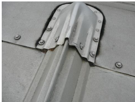
WIRE PROBE USAGE TO CHECK FOR SEALANT.
