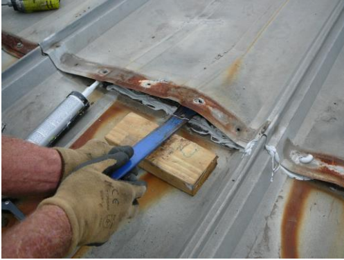
RESEALING END LAP WITH POLYURETHANE SEALANT.
