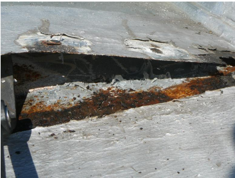
TRAPPED MOISTURE CAUSED ACCELERATED CORROSION.
