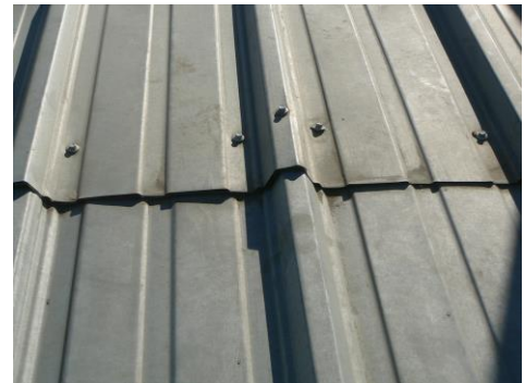
GAP BETWEEN ROOF PANELS AT END LAP.
