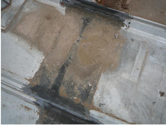
EPDM MEMBRANE REPAIR OVER A ROOF PANEL END LAP.
