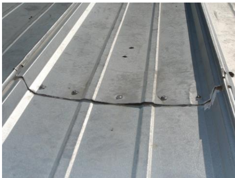
GAP BETWEEN ROOF PANELS AT END LAP.
