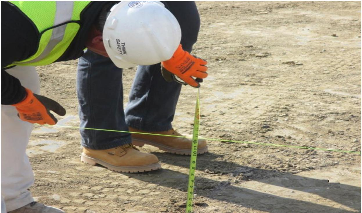
**VERIFY ELEVATIONS OF GRADE FROM STRING LINE REFERENCED FROM GRADE STAKES.**
