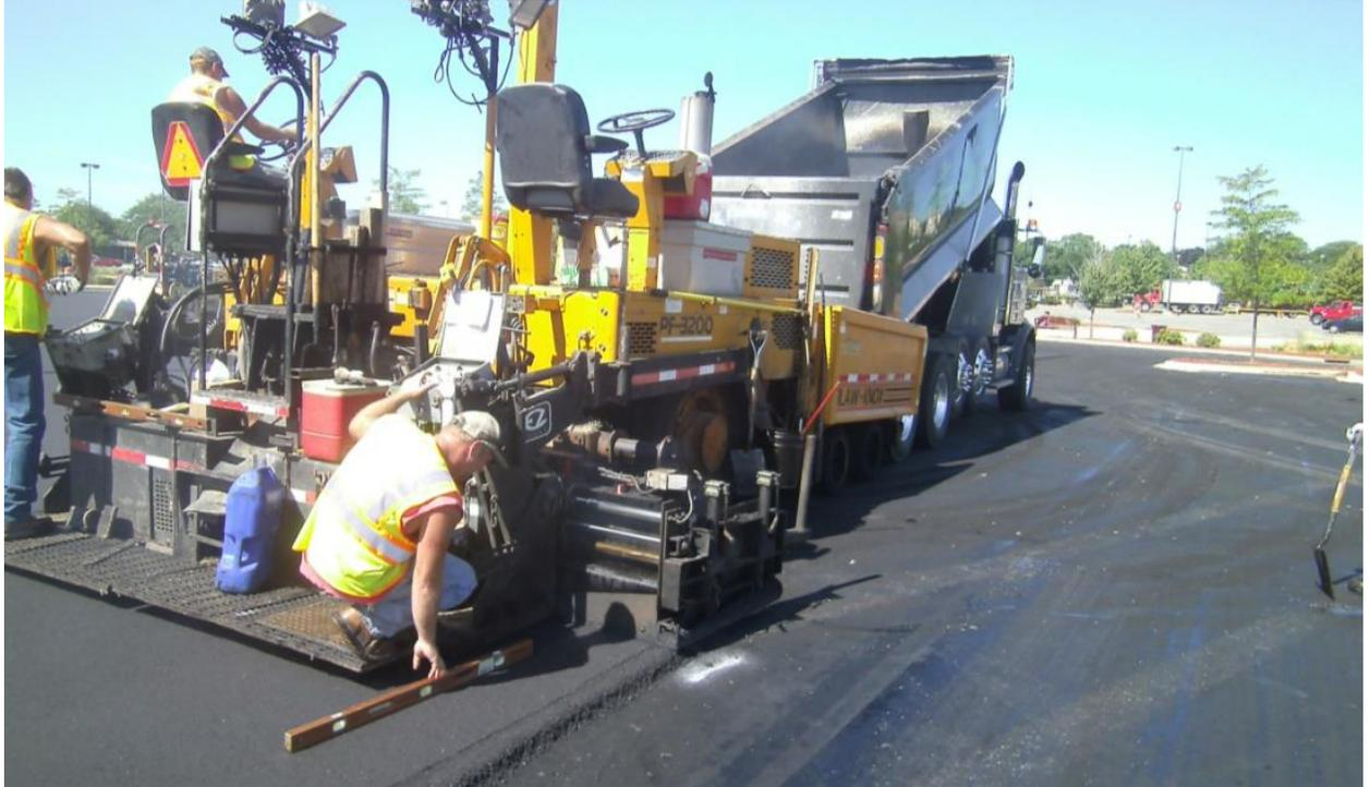
**CHECK ASPHALT PAVEMENT SURFACE SLOPE DURING PAVING OPERATIONS.**
