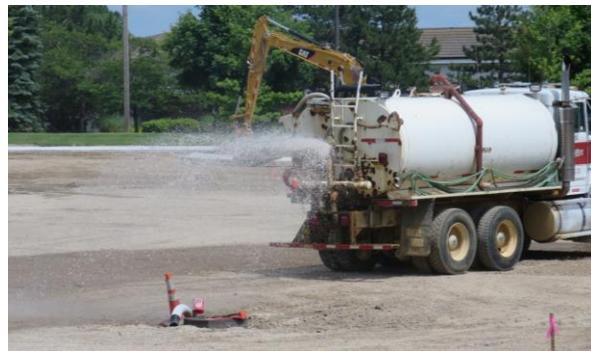
**WATER TRUCK APPLYING WATER TO AGGREGATE BASE TO AID WITH COMPACTION EFFORTS.**
