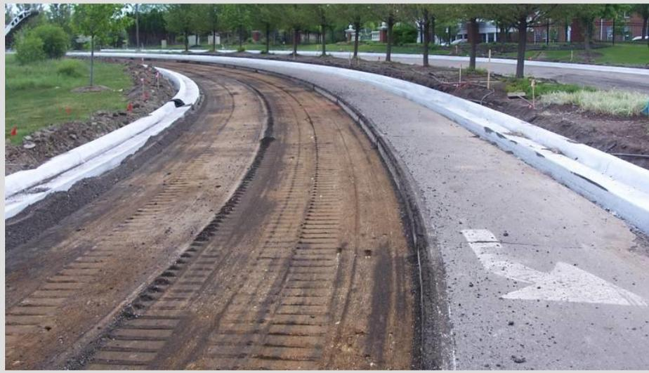
**Pavement removal by milling can minimize disruption to the grade and be more efficient, saving time and cost.**
