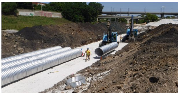
Drainage Pipe Installation
