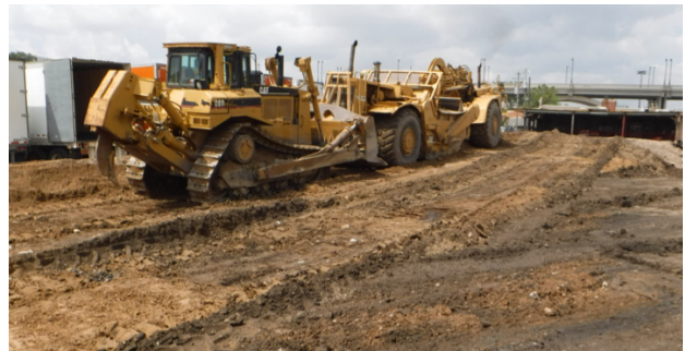
Sitework and Grading Preparation
