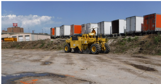
Prior to Construction
