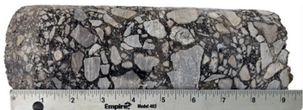
Multiple Asphalt Lift Core Sample
