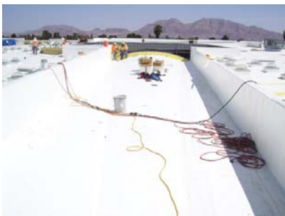
Overview of roof membrane installed.
