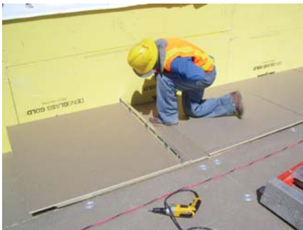
Rofer checking tapered board for insulation slope.
